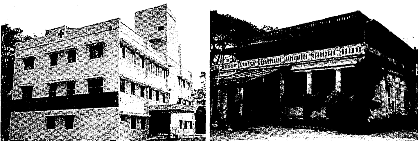
The new Dewan Bahadur Thatikonda Namberumal Chetty Day Hospital at the IRCS campus... and, right, the facility that existed in an old house here. (Text and photographs by RAJIND N CHRISTY.)
